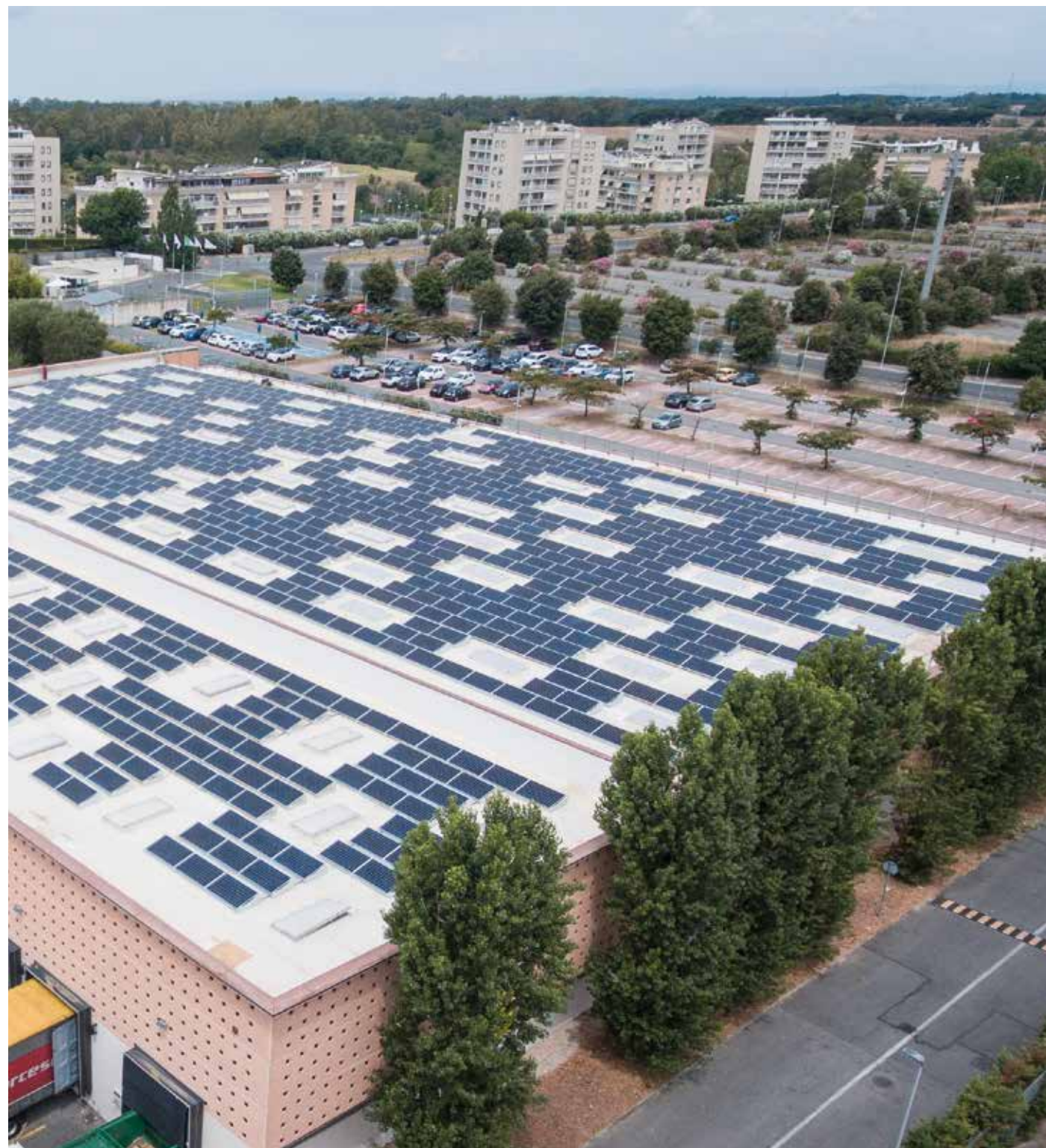
TMI's Parts Logistics Warehouse - The photovoltaic system installed on the roof produces 25% of the energy used in the Toyota Motor Italia headquarters.
